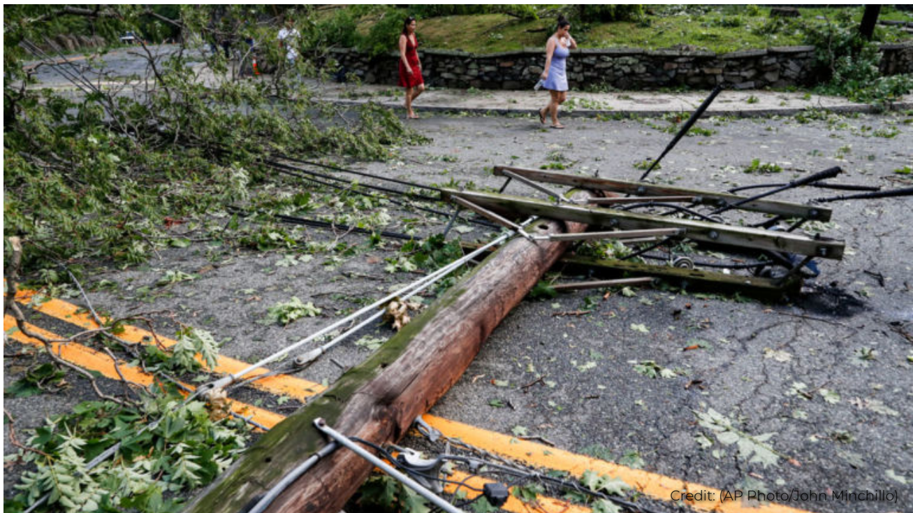
Power lines brought down in Edgewater during Tropical Storm Isaias
