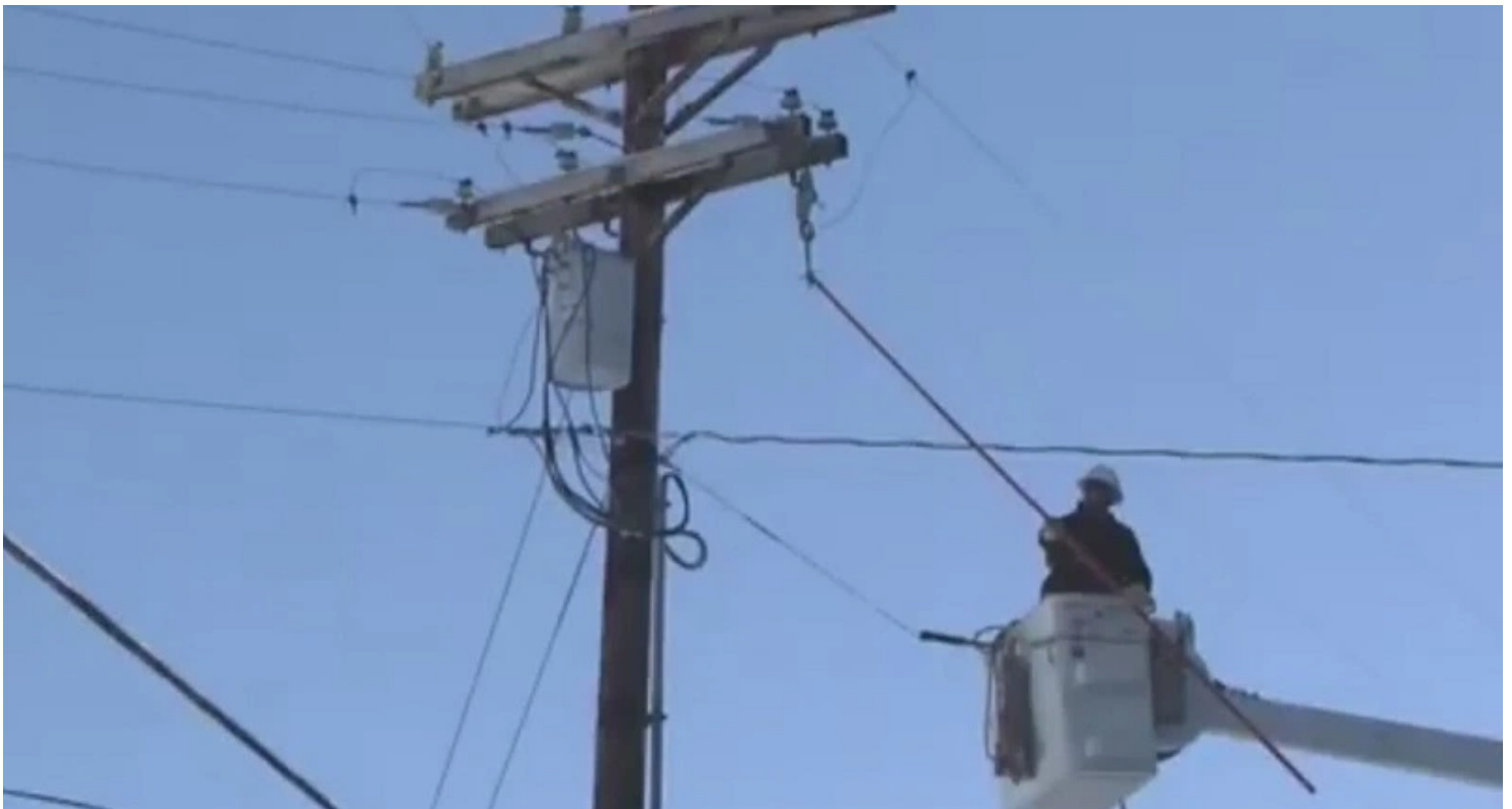
A PGE crew member repairing power (PGE, file)
