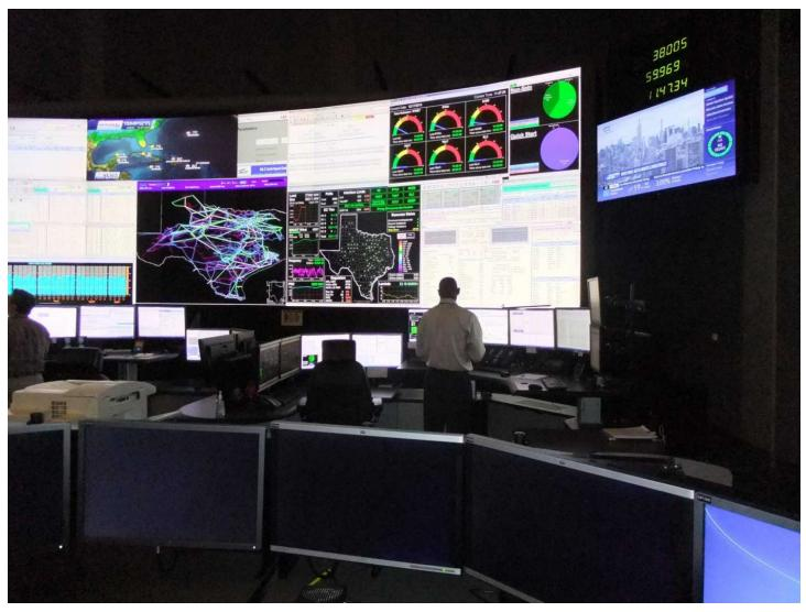
Workers in in the control room of the Electric Reliability Council of Texas, which operates most of the state's power grid, must keep a balance between electric generation and demand to prevent transmission lines from overloading. Ryan Holeywell / Houston Chronicle
