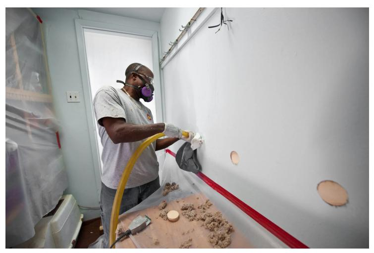
A worker blows cellulose insulation in the interior walls of a home. Credit: Dennis Schroeder / NREL
