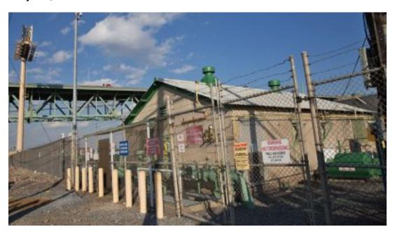
One of 9 Philadelphia Gas Works 'gate stations'. The gate stations are entry points where natural gas is regulated and depressurized before being pumped into the PGW network of pipelines. (Lindsay Lazarski/WHYY)
